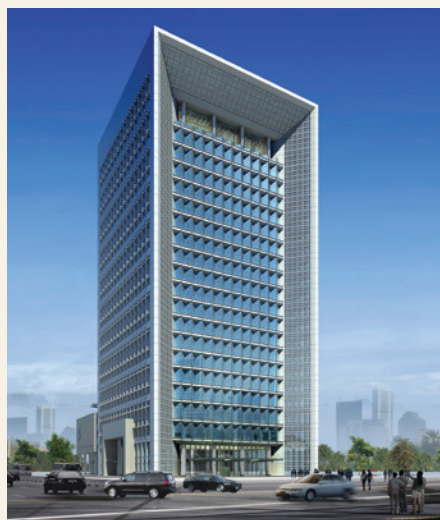
XIONG DUOKUI, ZHANG JUN, SUZHOU GOLD MANTIS CURTAIN WALL CO., LTD.
